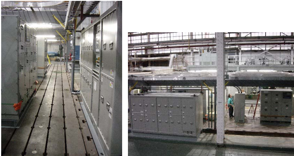
RCT Systems PCMs installed at Navy LBTS
